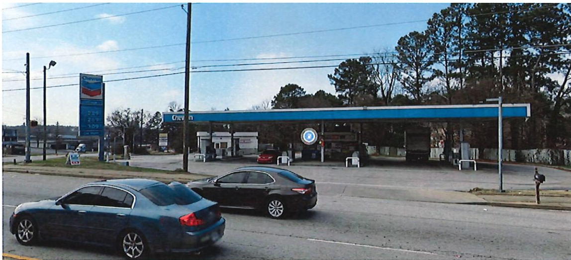
Figure 2: V22-000004 2799 Evans Mill Road
